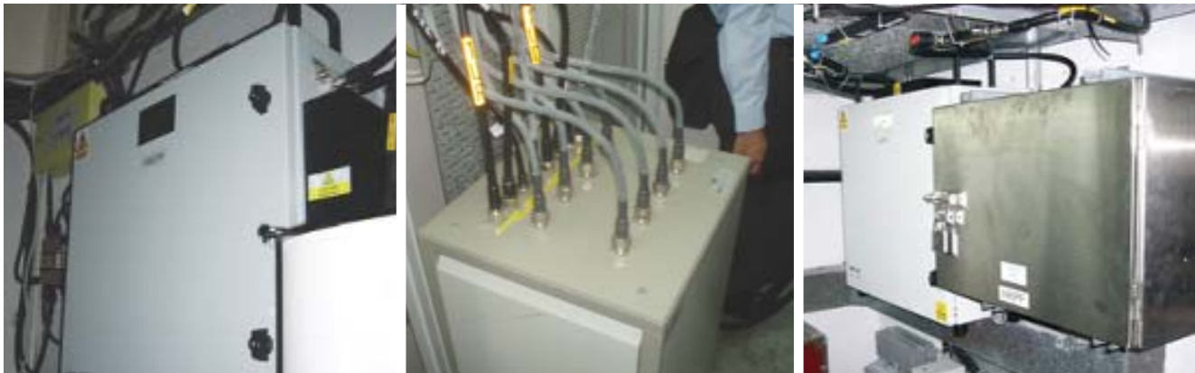
Equipment from the distributed antenna system (DAS), including bidirectional amplifiers, at Telford Plaza, a Hong Kong shopping mall.
